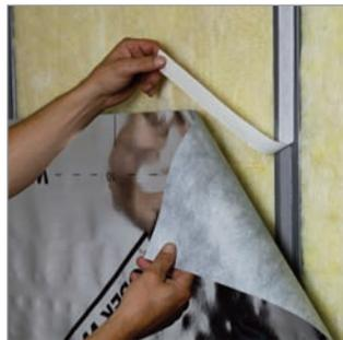
Butylon is a double-sided tape for sealing nail penetrations through underlays as well as sealing underlays, air barriers or vapour control layers (AVCL's) to both smooth and rough surfaces. Both internal and external use.
